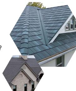
For example, if you live in a high-wind area and see a lot of your shingles blowing off your roof, you should take a good look at metal roofing. Because of the way it is made and installed on the roof, metal roofing will have fewer issues in blowing off your roof during high winds.
